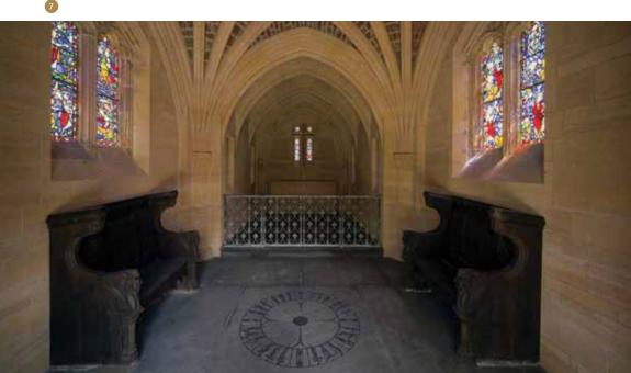
The interior walls of the chapel are Mankota stone, smoother than the exterior walls, striated by hand in alternating patterns. The walls are 20 inches thick: 12-inch exterior walls, a four-inch air space, and four-inch interior walls.
